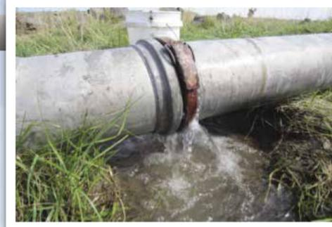
This photo shows a leaky gasket (or absent gasket?) at a mainline joint. Due to volume of the pipe, it loses 24 gpm at 50 psi. If lifting water from a 30-foot drop (like a canal system) losses would total \$111 per year just in electrical fees. If pumped from a well 300-feet deep, electrical fees would equal \$318 per year, and water losses will equal 6.62 acre feet.
